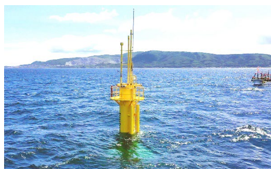
Floating structure in place
