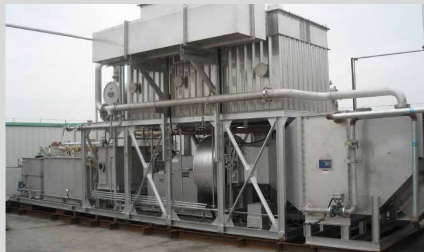
VOC treatment system [K-FILTER™ VOC Recovery Equipment]
